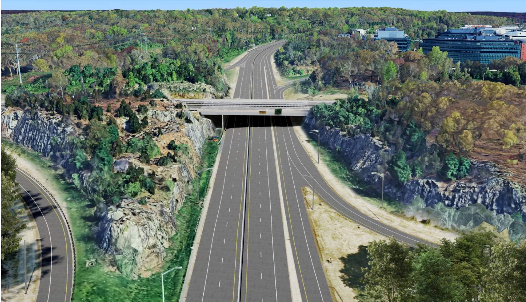
Route 7 Aerial View looking North
