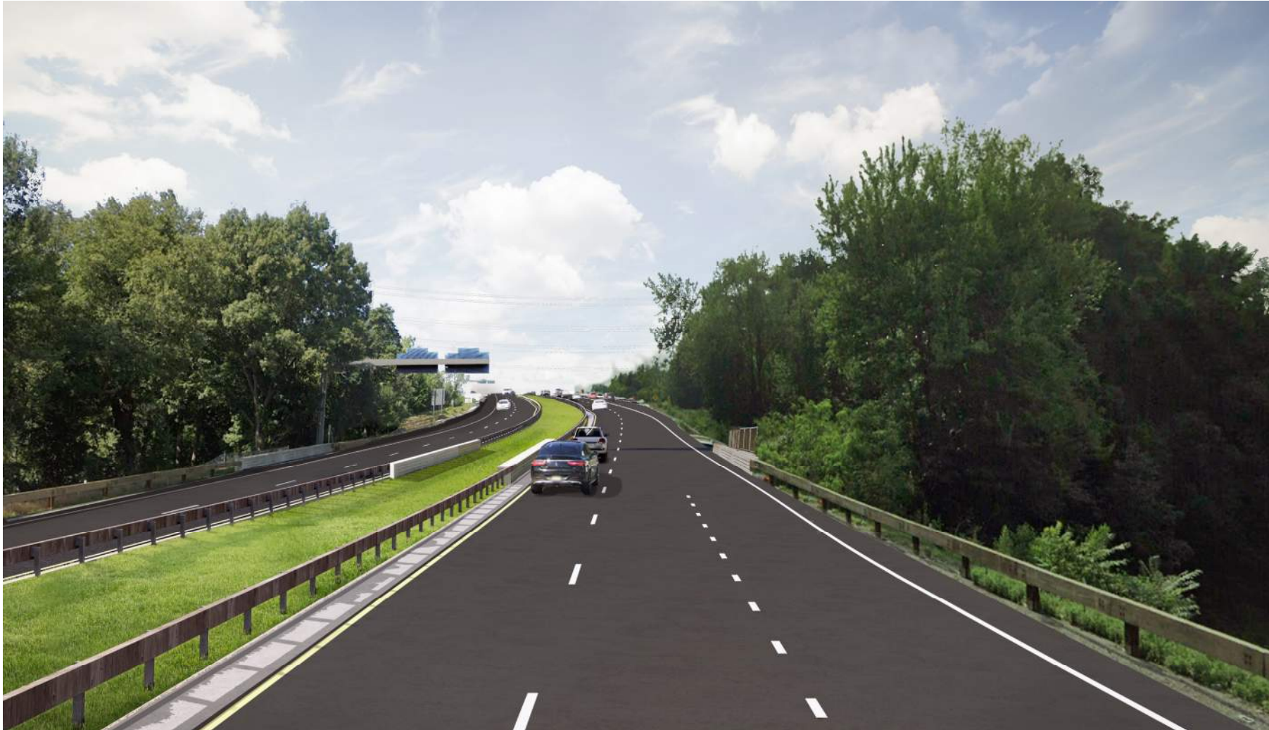
Route 15 (Merritt Parkway) view southbound at Metro North Railroad bridge
