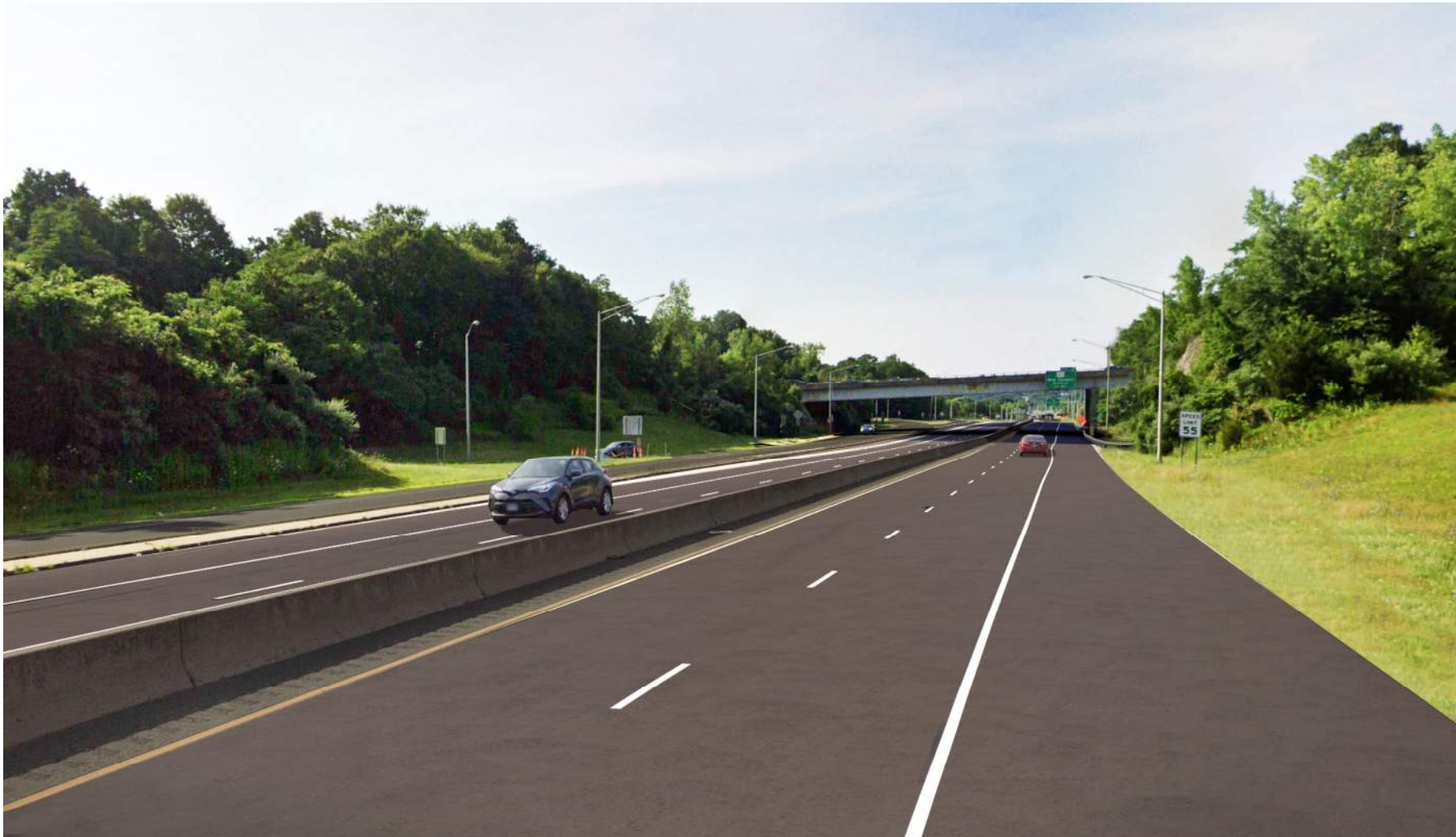
Route 7 street view looking South
